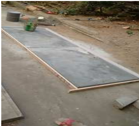
Mould for the construction of wall panel
